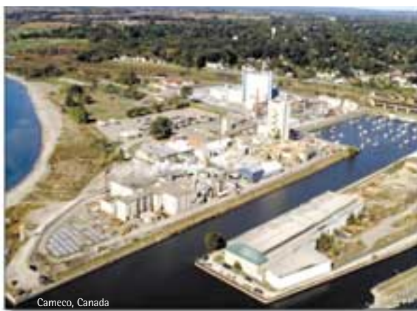
The uranium conversion facility at Port Hope, Canada, and the surrounding residential community.
