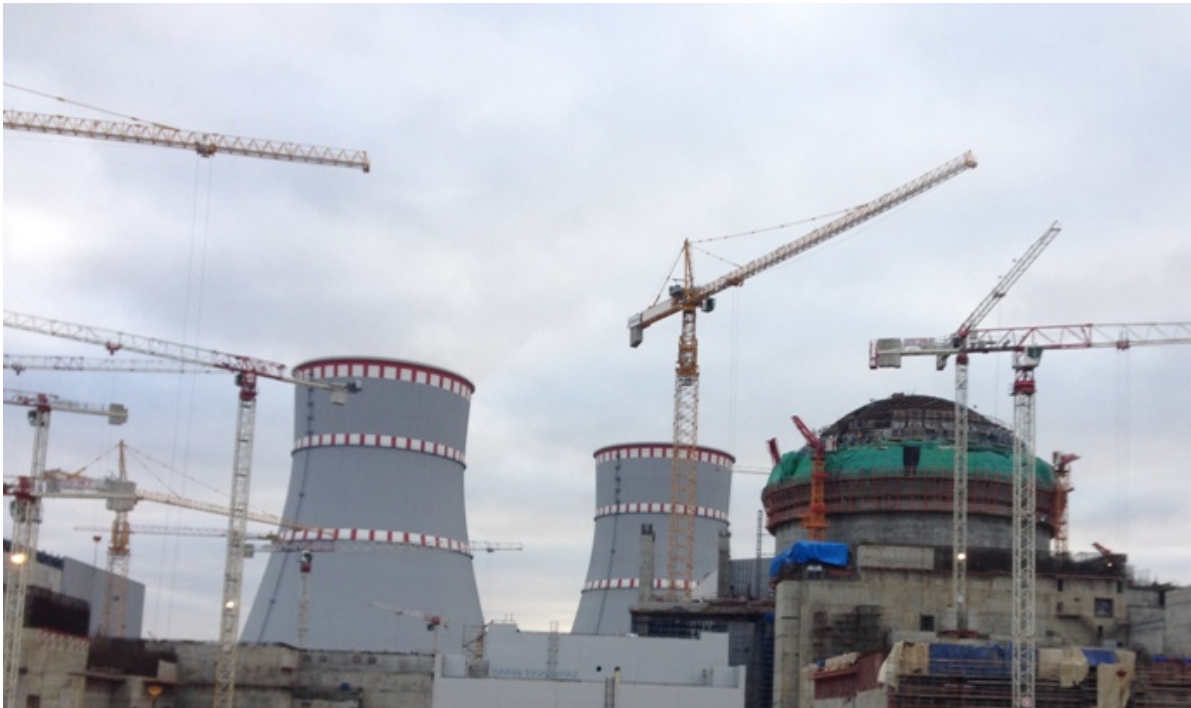
Leningrad 2 – Overview of the construction site, VVER, Russia, September 2014.
