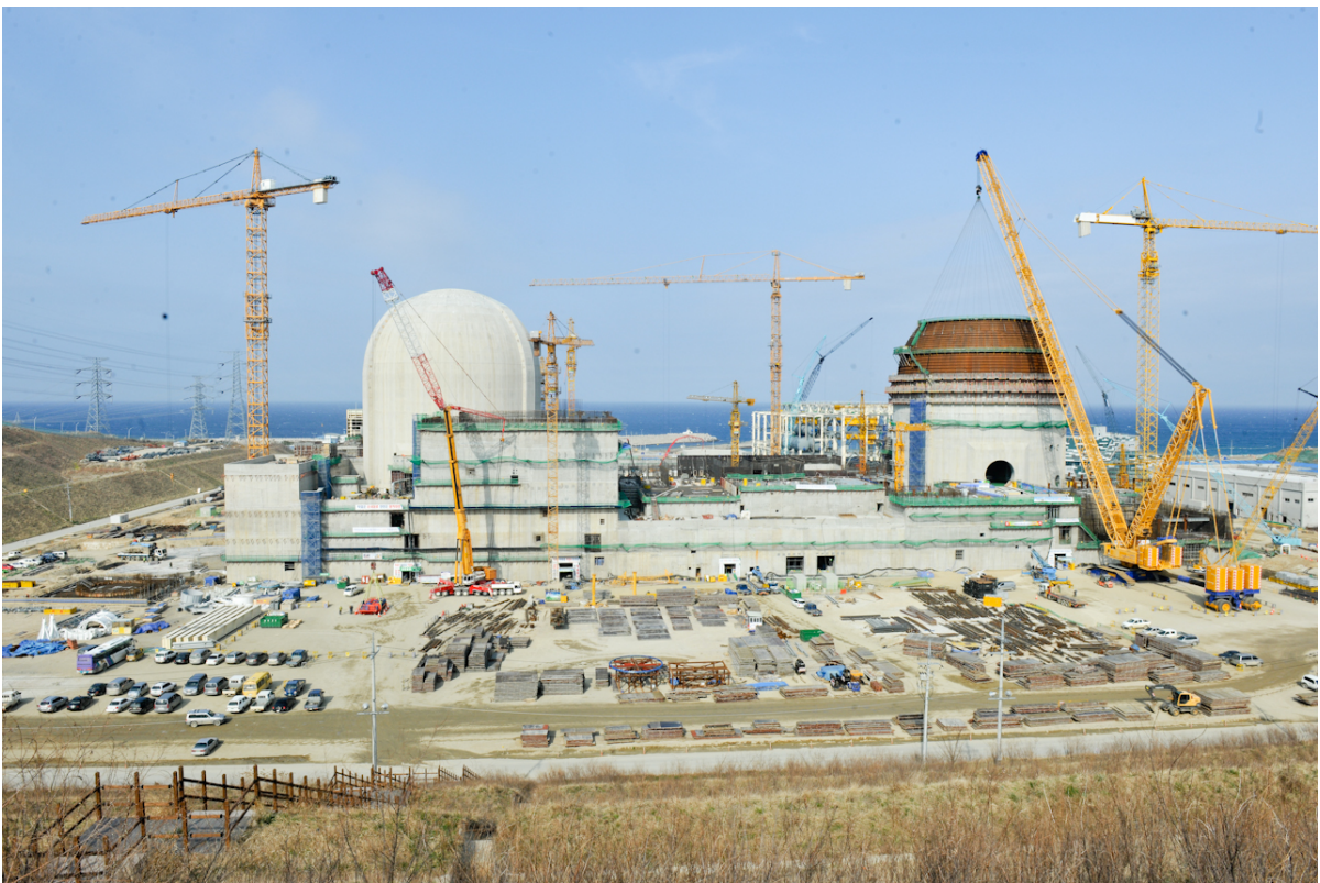
Shin Hanul – Construction site overview, APR1400, Korea, 29 March 2015 (provided by KINS).
