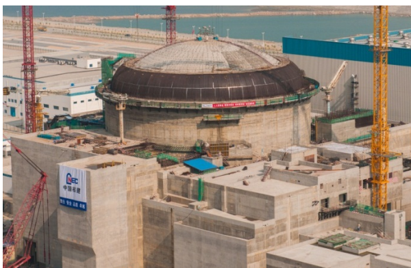
Taishan Unit 1 – EPR, China, September 2014. (provided by NNSA).
