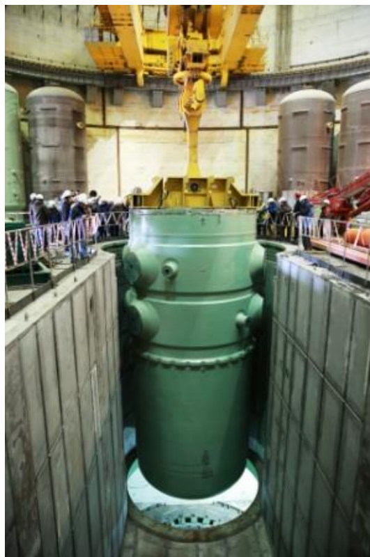
Novovoronezh 2 – Installation of Unit 2 reactor pressure vessel, VVER, Russia, 30 March 2015.
