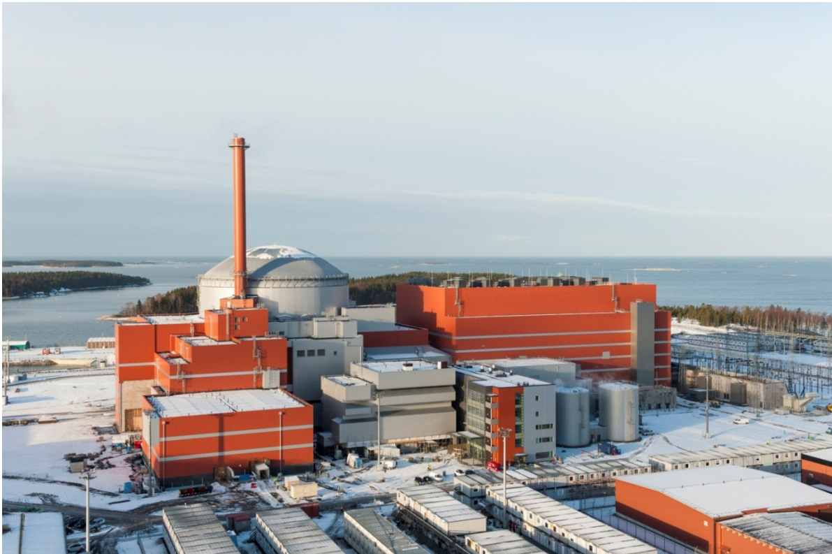
Olkiluoto 3 – Construction site, EPR, Finland, 23 February 2015 (Hannu Huovila/TVO).
