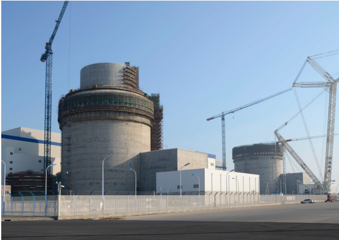
Haiyang Unit 1 – Construction site, AP1000, China, 13 February 2015 (provided by NNSA).
