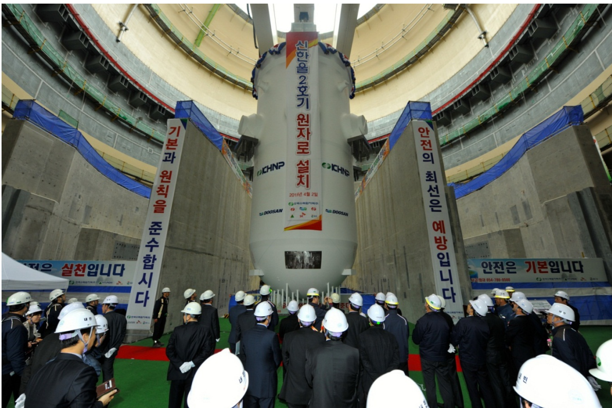
Shin Hanul Unit 2 – Setting of reactor vessel, APR1400, Korea, 2 April 2015 (provided by KINS).
