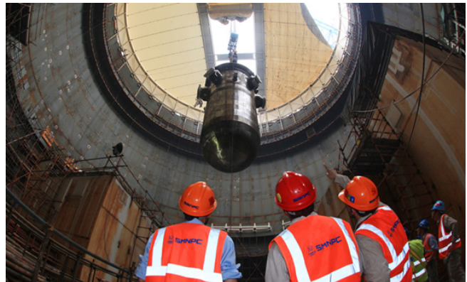
Sanmen Unit 2 – Reactor vessel hoisting, AP1000, China, 25 August 2014 (provided by NNSA).
