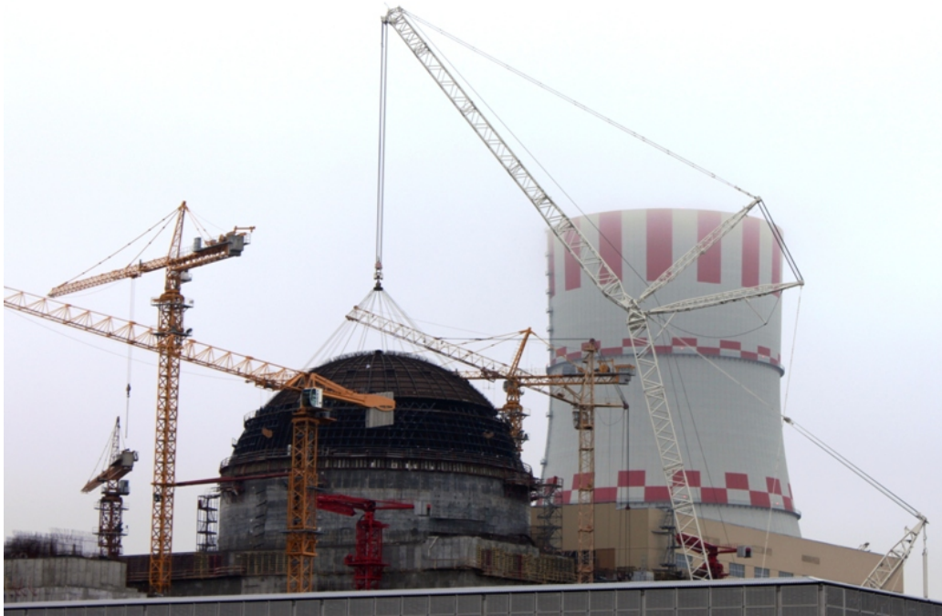
Novovoronezh 2 – Installation of the Unit 2 dome, VVER, Russia, 15 November 2014.
