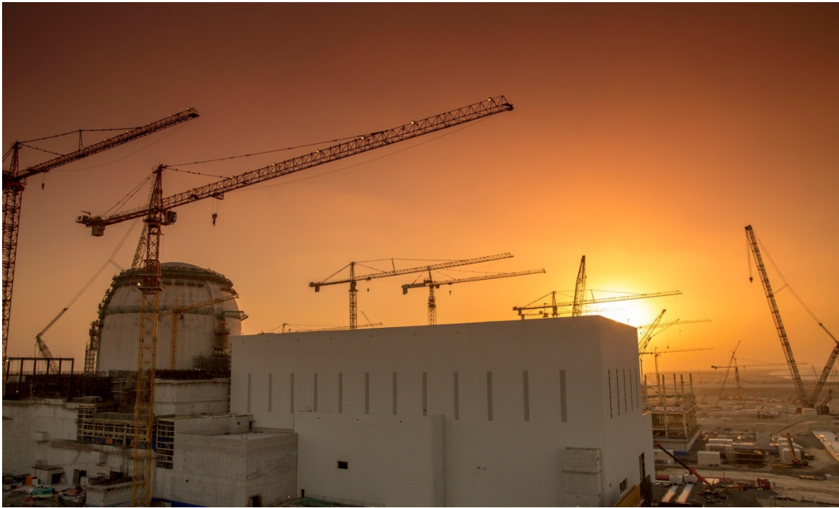
Barakah Unit 1 – Overview, APR1400, United Arab Emirates, 18 January 2015 (property of ENEC).
