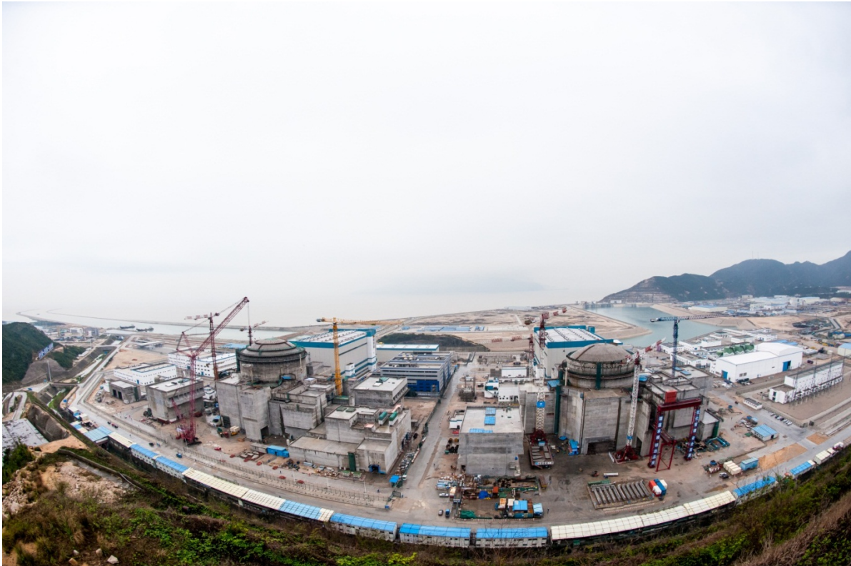
Taishan Units 1 and 2 – EPR, China, March 2015 (provided by NNSA).
