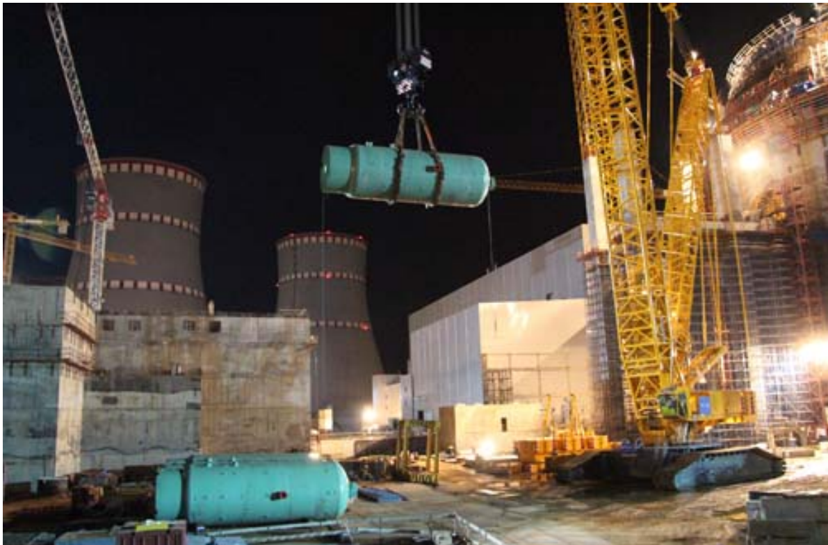
Leningrad 2 – Installation of the 4 ECCS accumulators, VVER, Russia, 9 October 2014.
