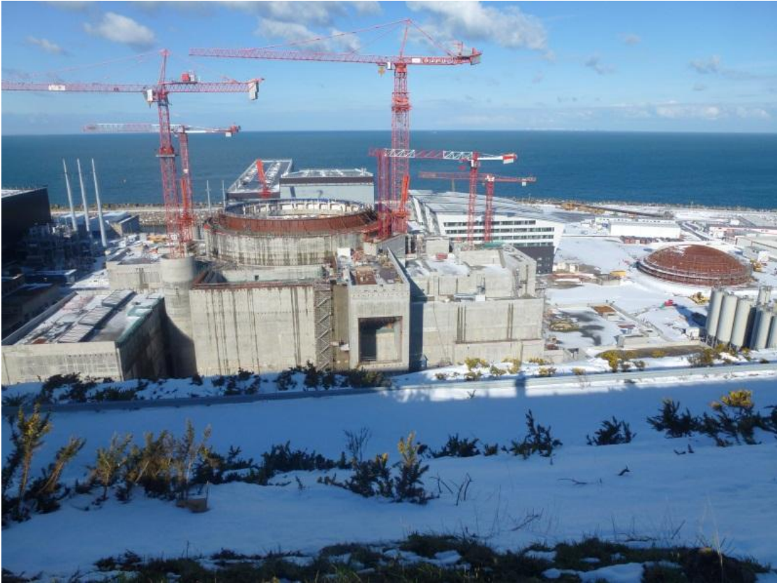
Flammanville 3 EPR reactor, France: March 2013. Copyright EDF.
