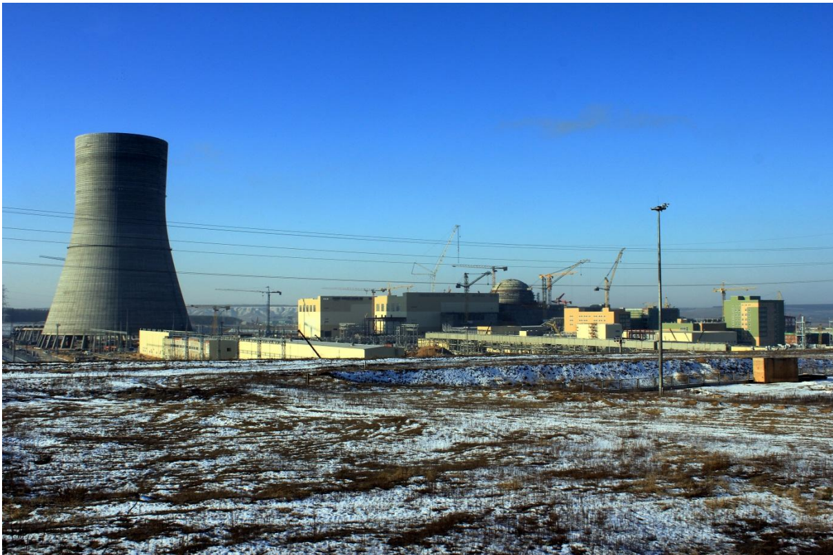
Novovoronezh VVER AES 2006 Phase 2, Russia: 2013. Provided by Rostechnadzor.
