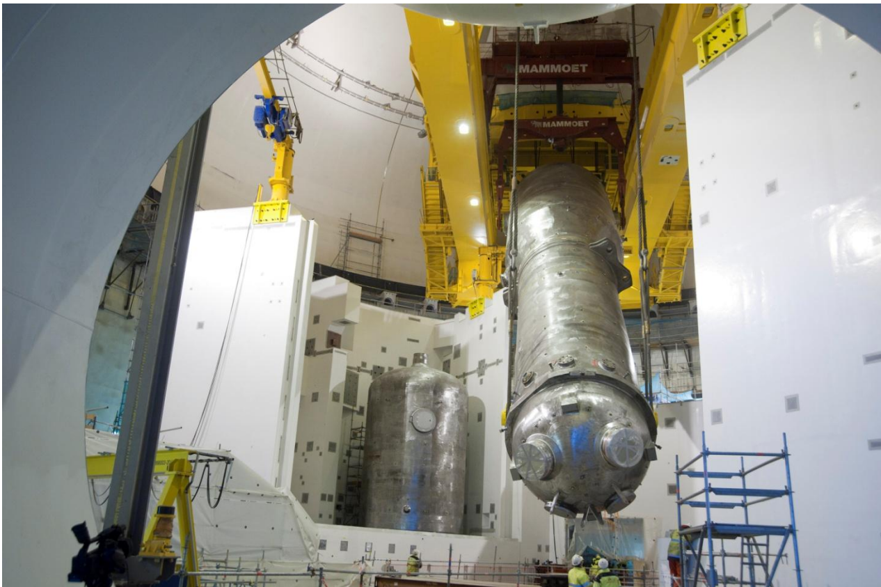
OL3 Steam generator installation; © TVO 2010.
