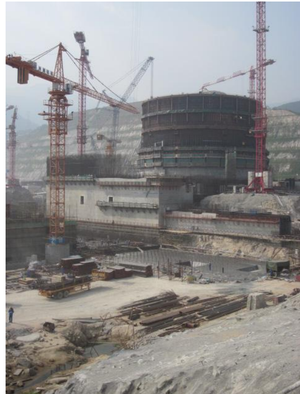
EPRWG site visit in Taishan (EPR under construction)
