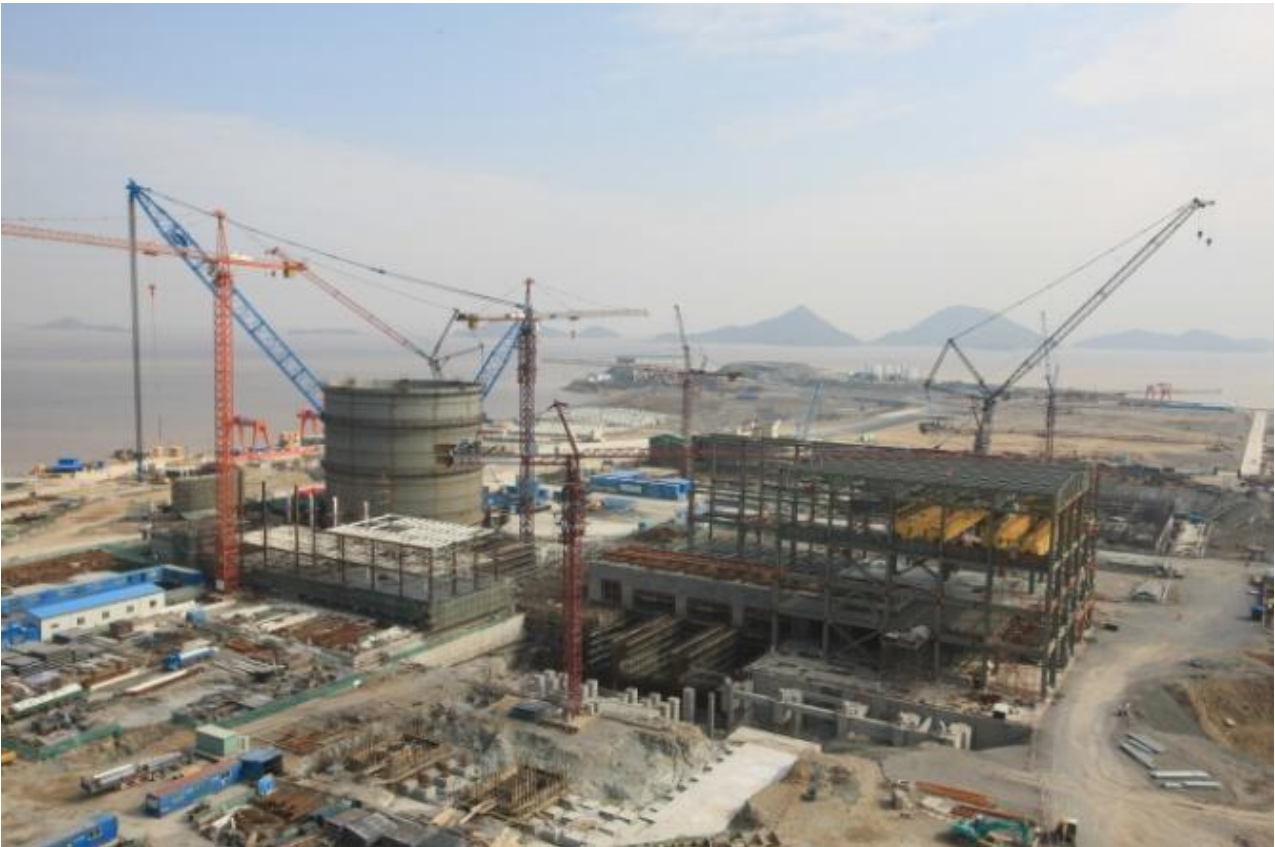
AP1000 under construction, Sanmen, China; © SNMPC 2010.
