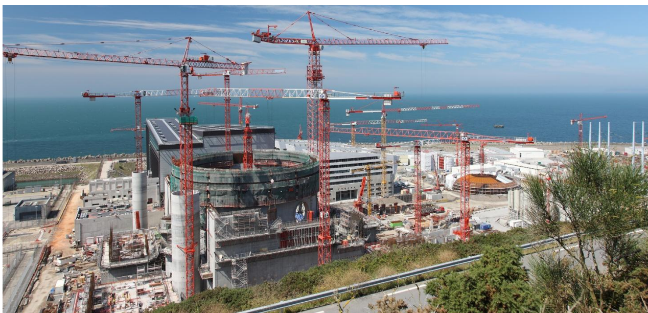
Flamenville 3 – Construction site -© EDF
